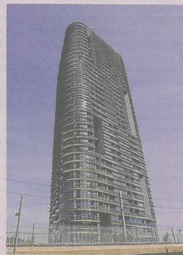
Problems continue for owners Opal Tower apartments. PHOTO: AAP
